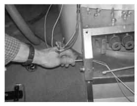
Step 13: Pull pilot wires through burner box
